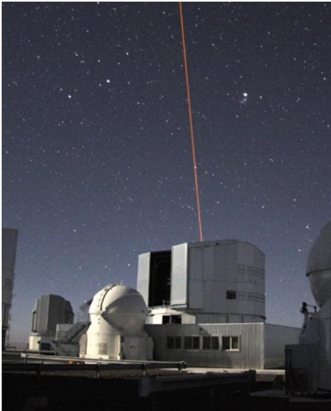
**FIGURE 7: A 50-cm wide yellow laser beam is coming out of ESO's Very Large Telescope (VLT) in Chile. The laser light illuminates Sodium atoms located in the upper atmosphere at 90 km altitude and creates an artificial star. The laser guide star (LGS) is analyzed by Shack-Hartmann wavefront sensors and used to optimize the adaptive optics of the telescope mirrors. (Image by Sylvain Oberti, ESO)**
